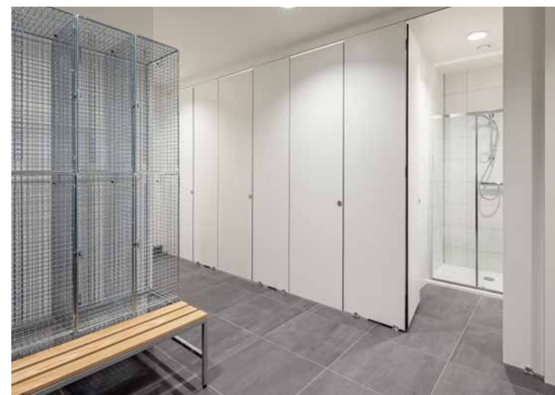
Landmark showers, lockers and changing rooms
