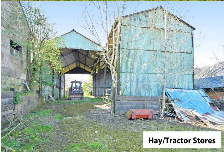
Brick Built Barn with Stable and Loft over
