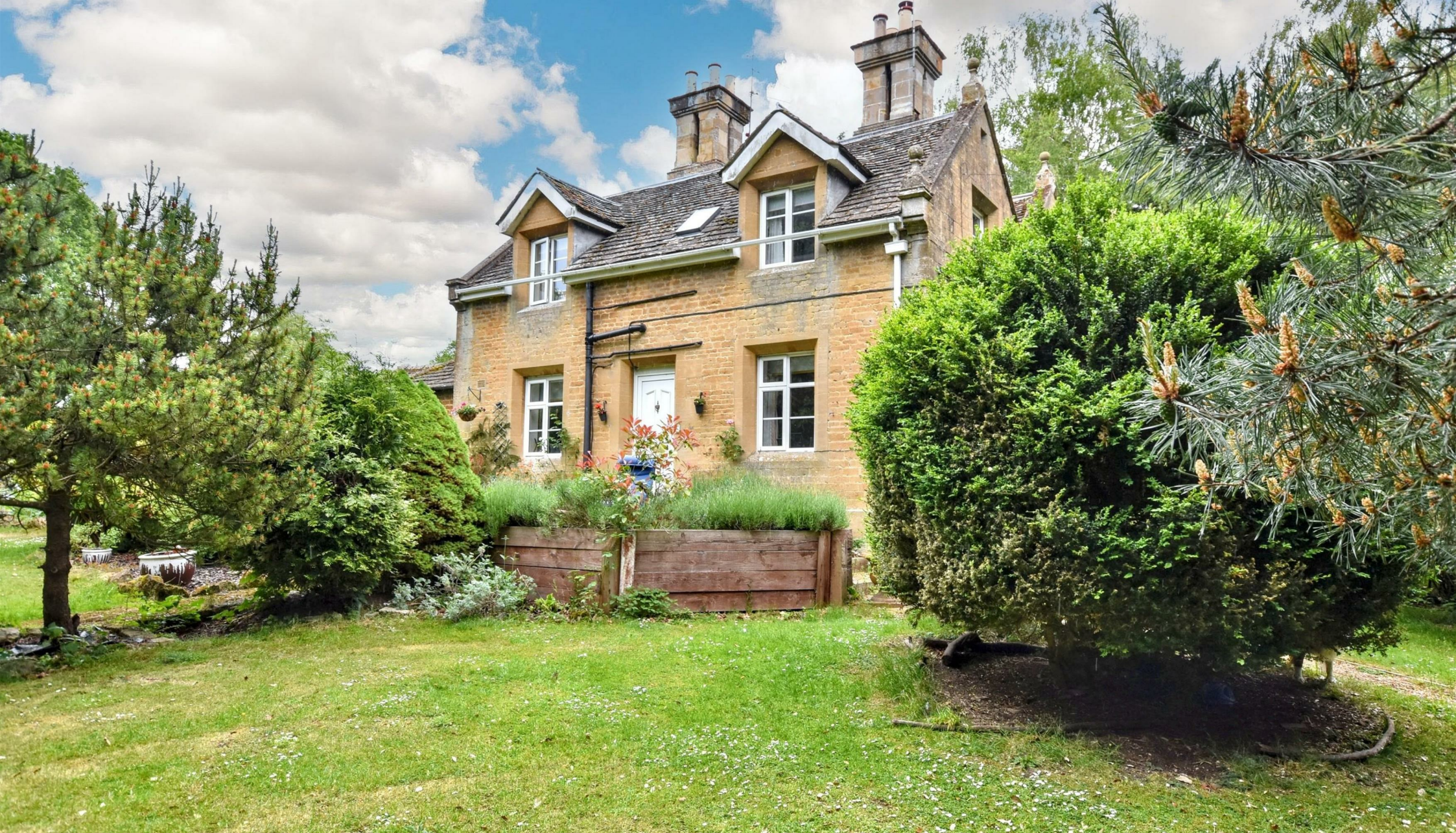
Park Cottage Willow Brook Road Corby, NN17 2UG
