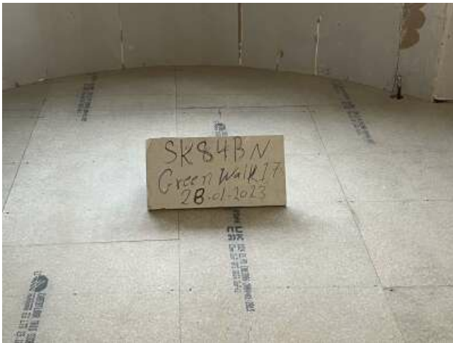
Installation of 22mm wood floorboard in second floor
