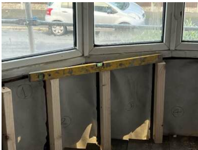
Installation of 22mm chipboard in first floor
