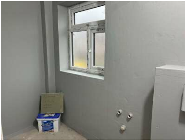
Installation of Mapei Waterproofing membrane
