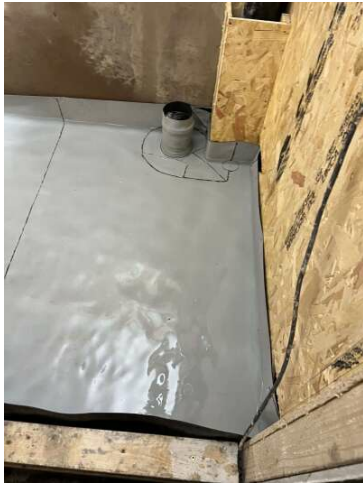
Installation of Mapei Waterproofing membrane
