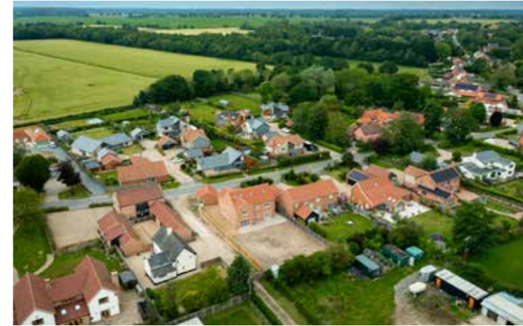
Aerial view of the property
