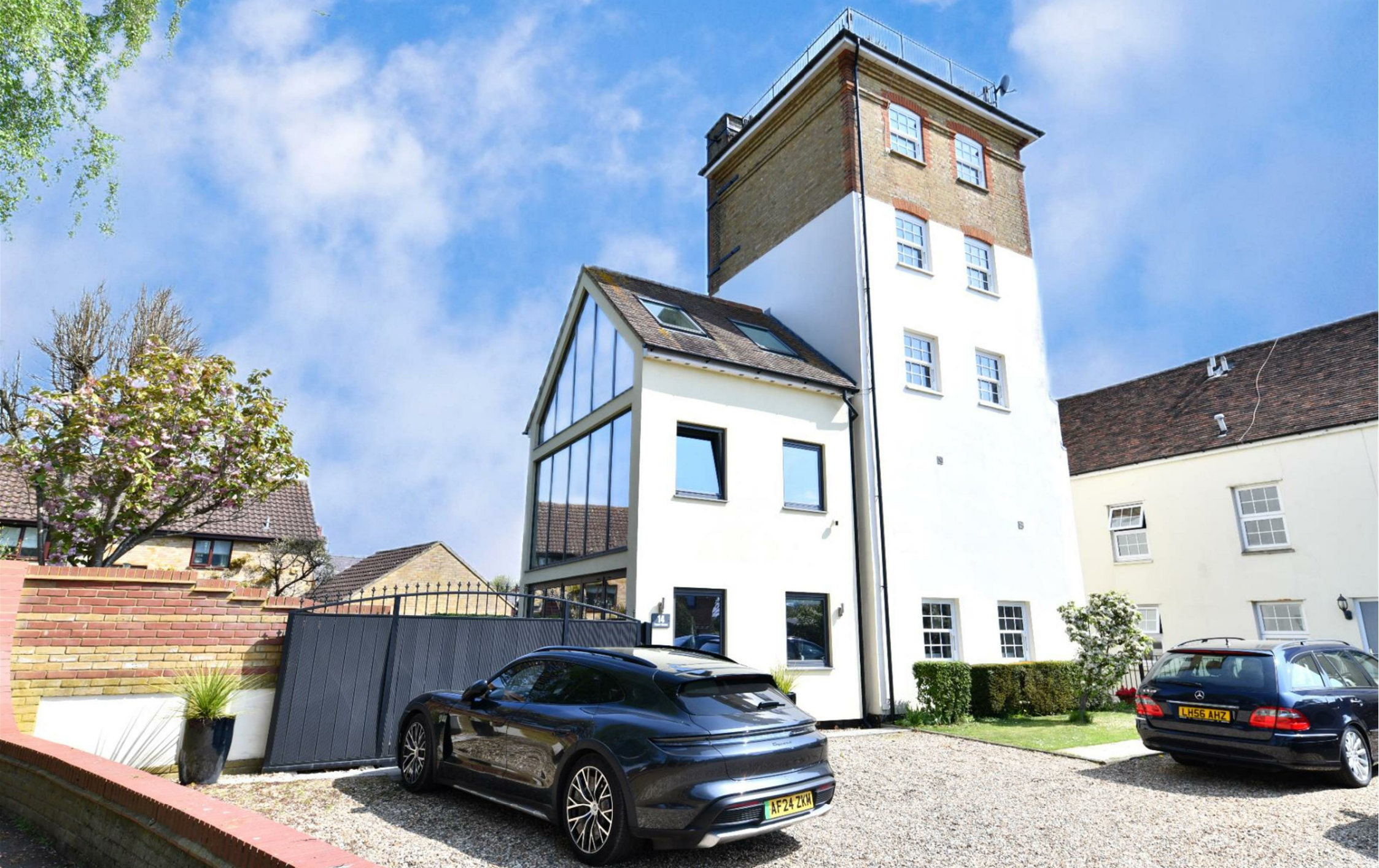
The Maltings, Walkern, Stevenage
