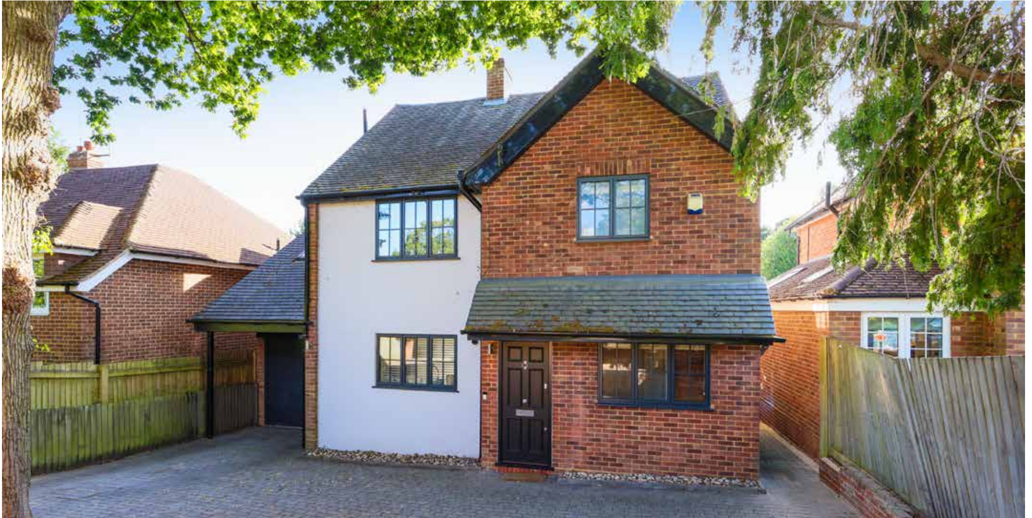
CHAUCER AVENUE, WEYBRIDGE
