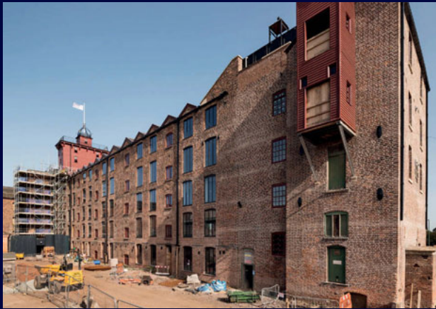
Back of the Main Mill during restoration © Historic England
