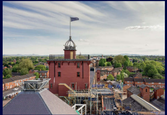
View of Jubilee Tower looking towards Shrewsbury town centre © Historic England
