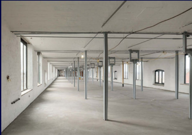
Third floor of Main Mill during restoration © Historic England
