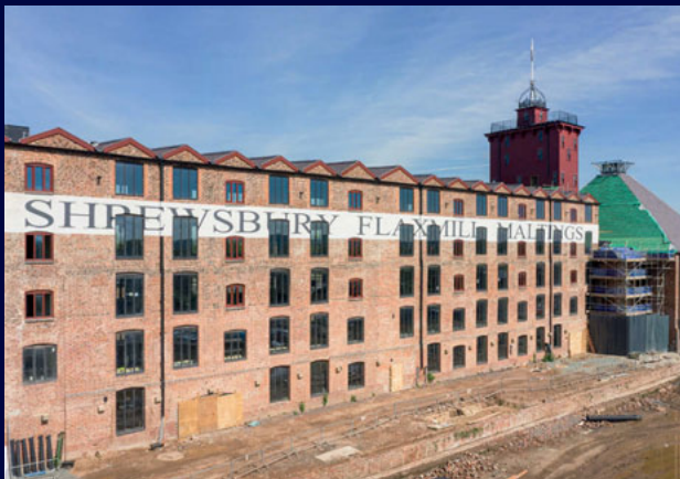
Front of the Main Mill during restoration © Historic England
