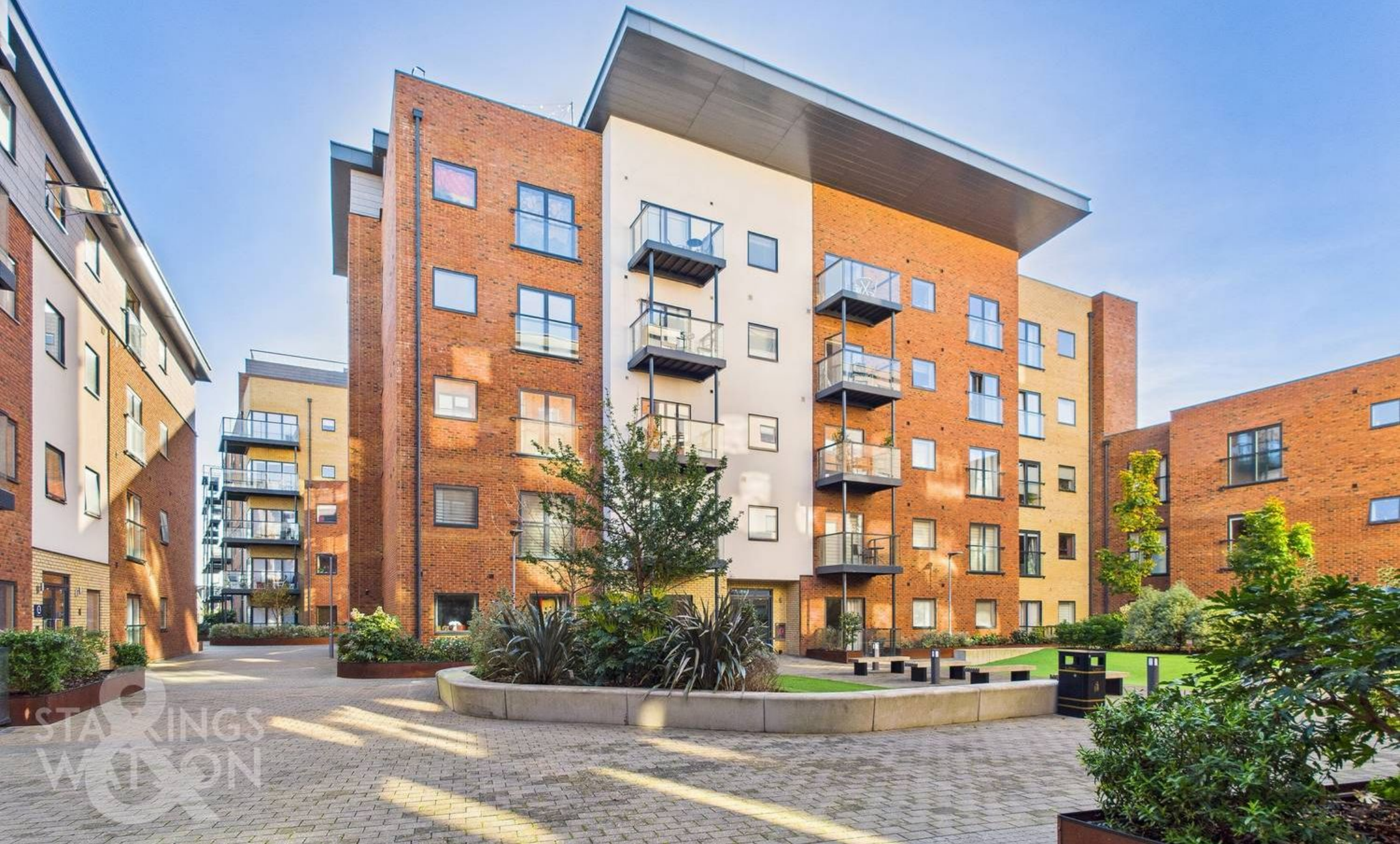
Austin House King Street, Norwich - NR1 1FW
