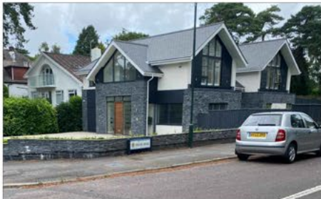
Image 3 - design intent new aluminum doors & stone cladding
