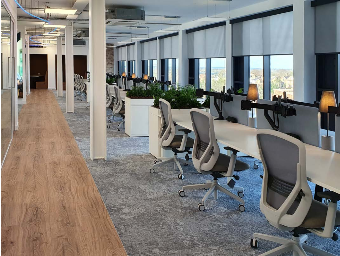
THE K2 CORPORATE MOBILITY FIT-OUT IN PROGRESS ON THE FIFTH FLOOR.
