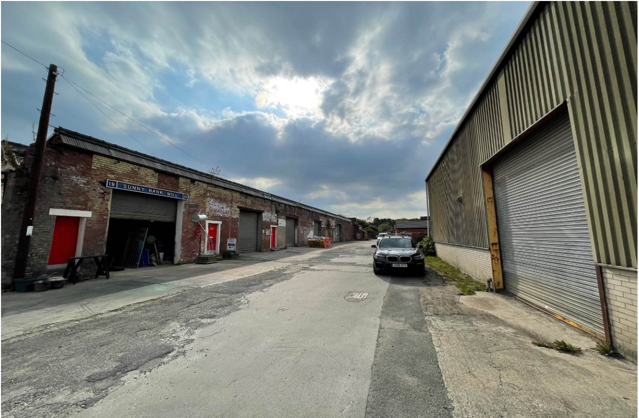
Entrance road into Sunnybank Mill site.
