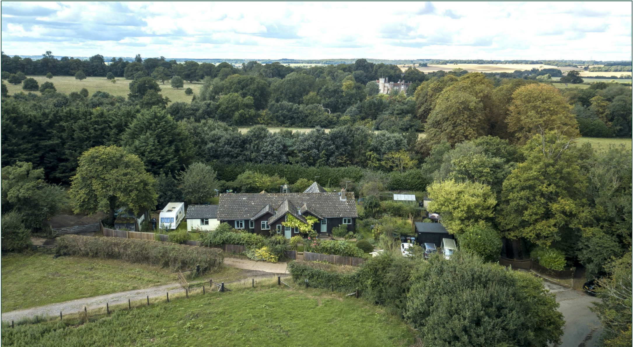
The Lodge Ardeley, Stevenage, Hertfordshire, SG2 7AF
