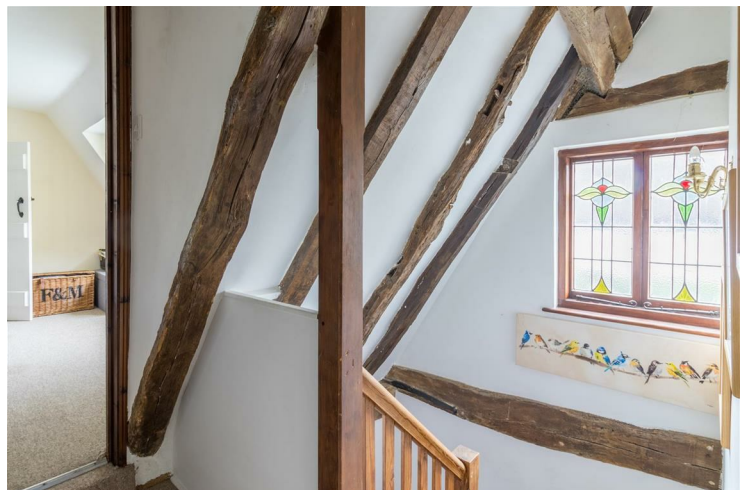
FIRST FLOOR LANDING
