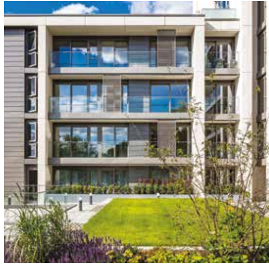
Tileman House, Putney
