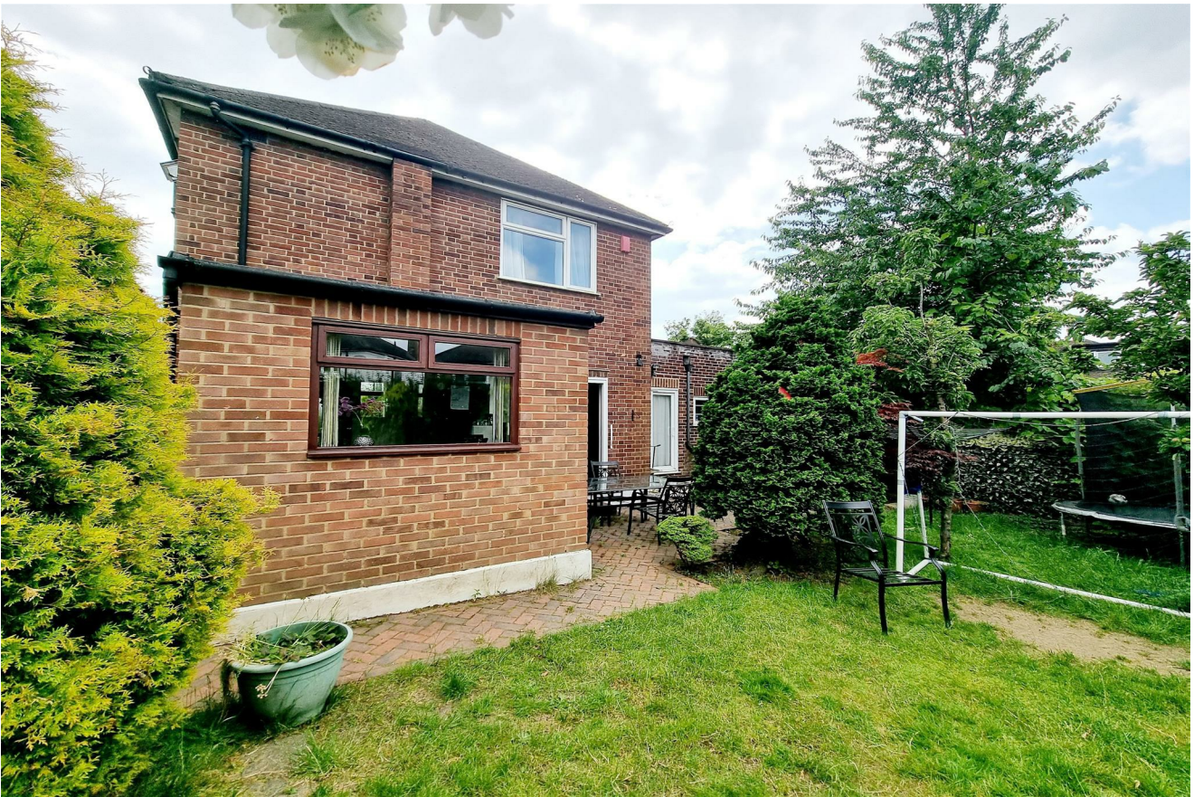
REAR ELEVATION OF PROPERTY: PIC. 2 Showing Annexe & Garage to Side.
