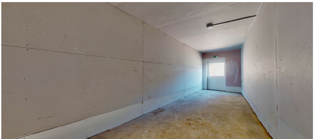
Interconnecting Rear Access with Main Unit
