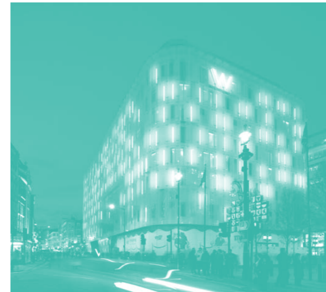
W London is a landmark 192 bedroom, 5 Star hotel in the heart of London's West End, developed by McAleer and Rushe, designed by Jestico + Whiles.
