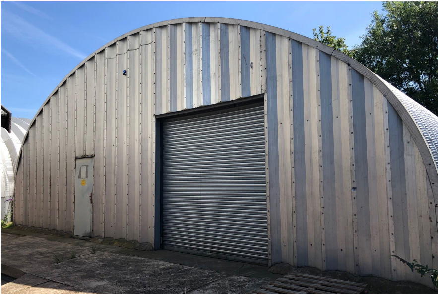
Rear Yard - External Workshop / Store
