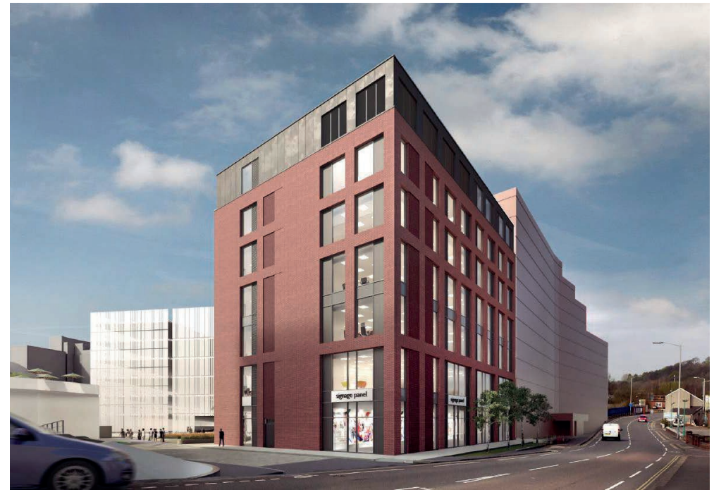
View of the offices from Brimington Road.
