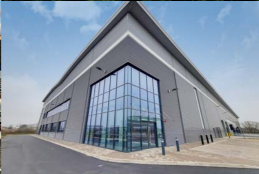
ASCENT LOGISTICS PARK LEIGHTON BUZZARD Eight warehouse / industrial units 14,140 to 123,490 sq ft - FULLY LET
