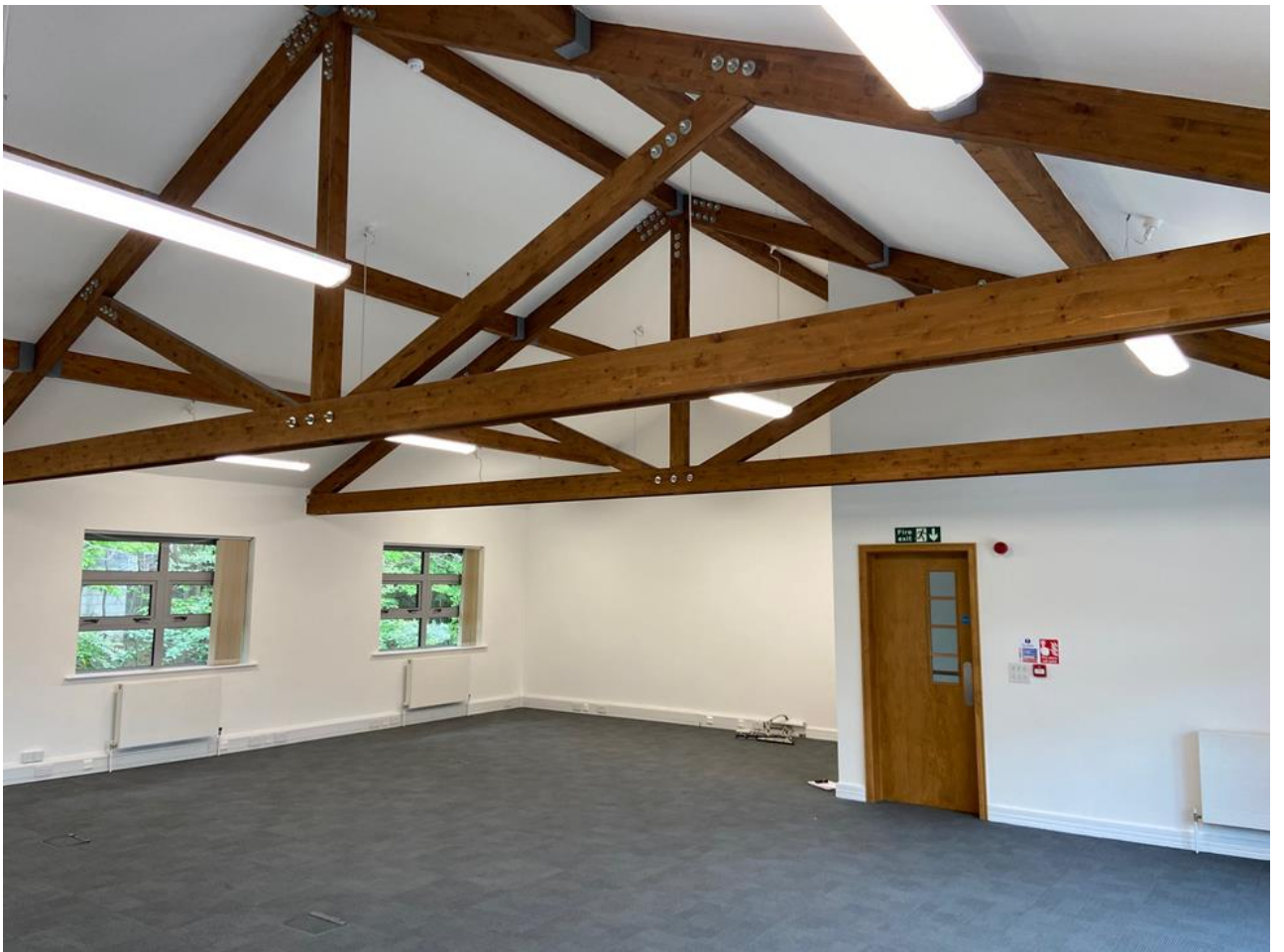
Images of Unit 9, Market Dock – the available units will be refurbished to the same specification.
