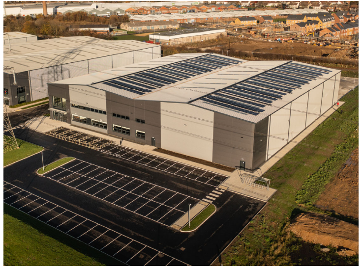
Completed Intersect 19 facility, North Tyneside
