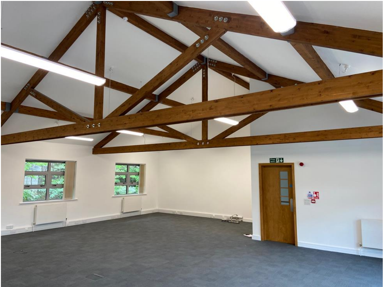
Images of Unit 9, Market Dock
