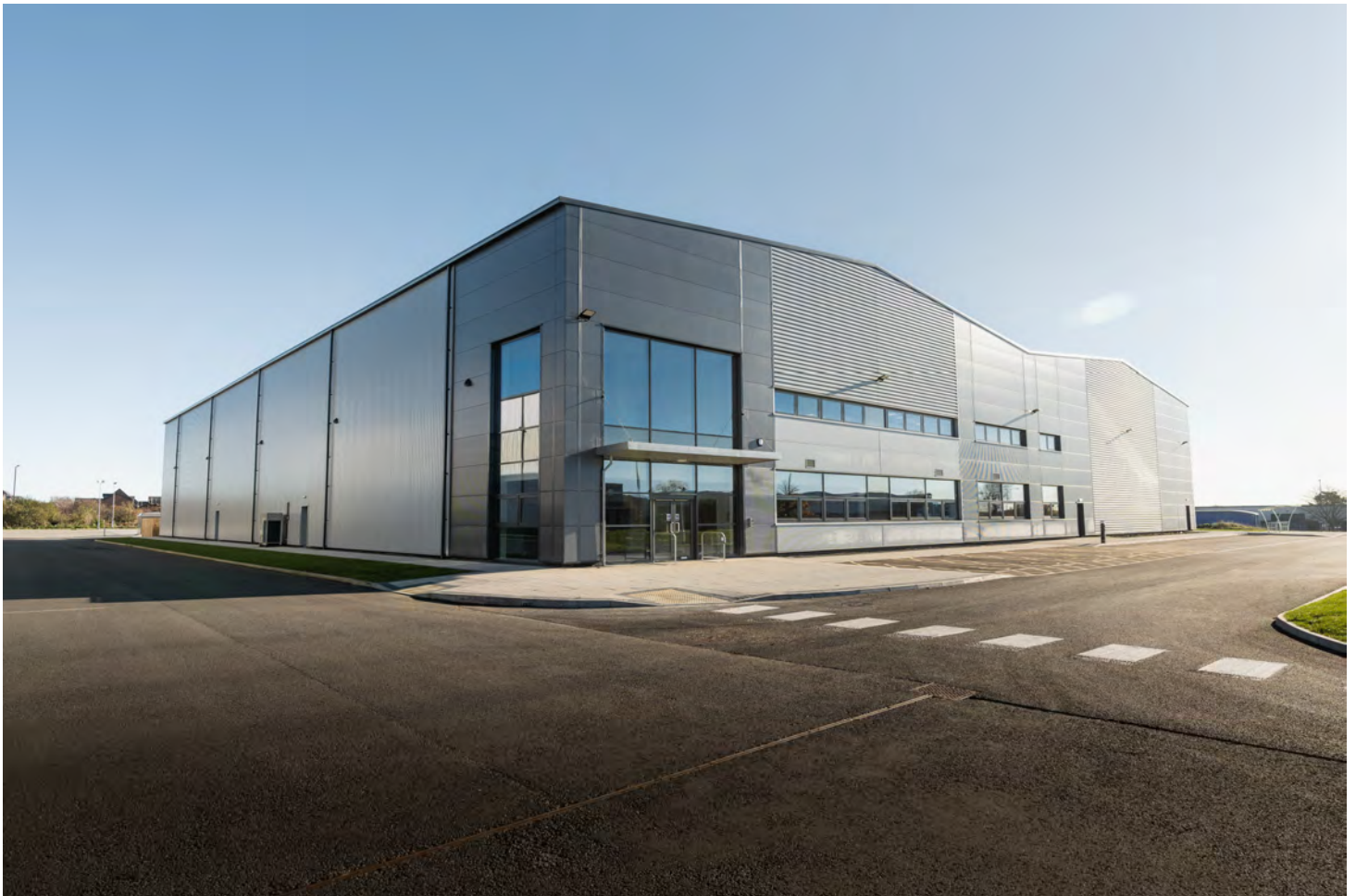
Image of completed Unit L6 (June 2023)
