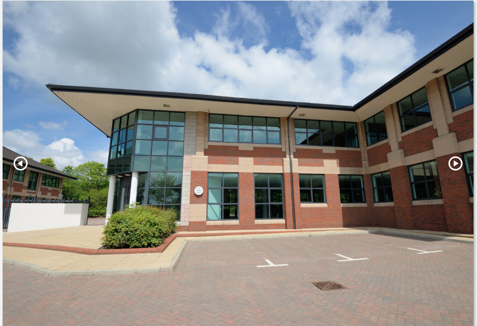
St Andrews House
