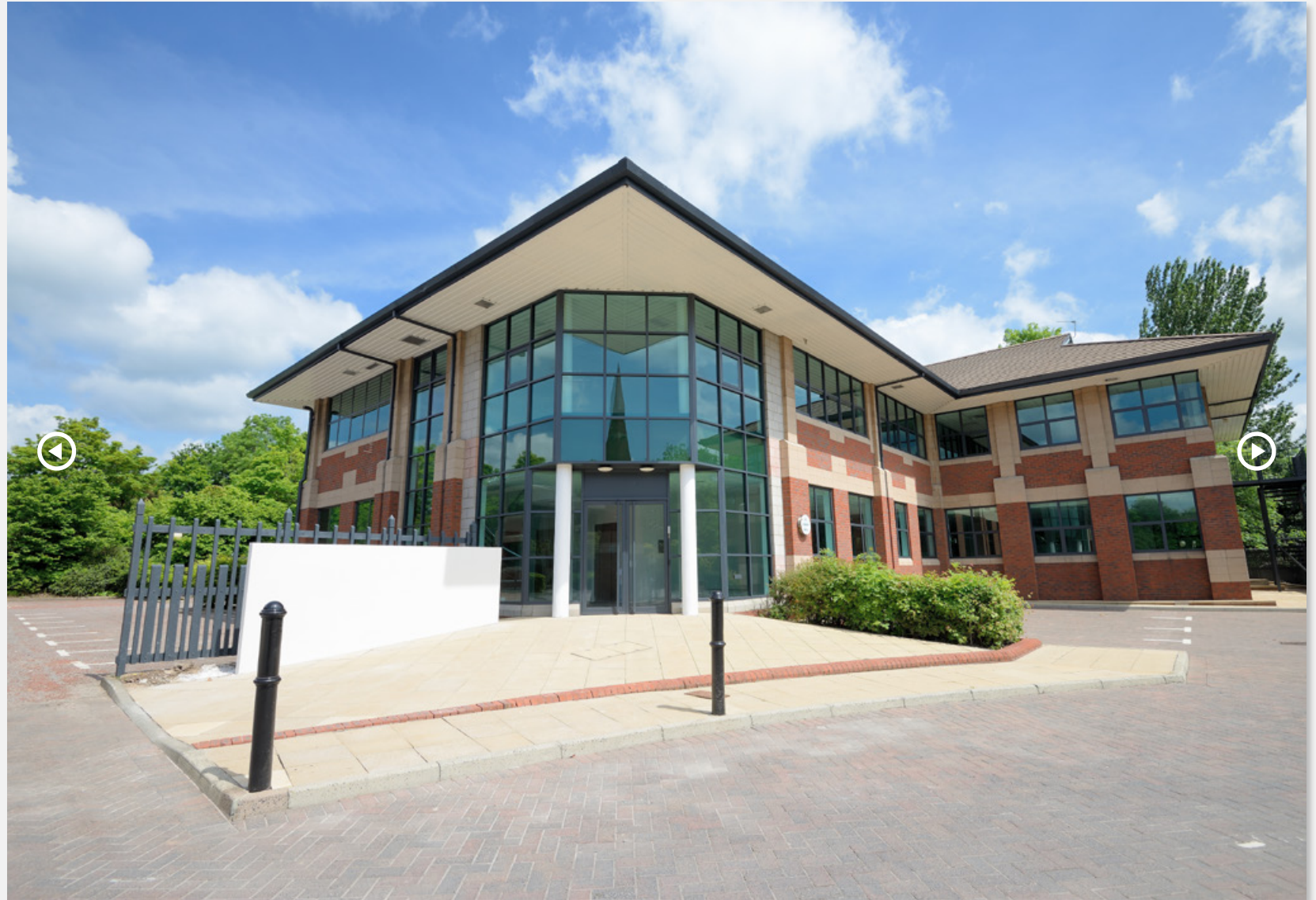
St Andrews House
