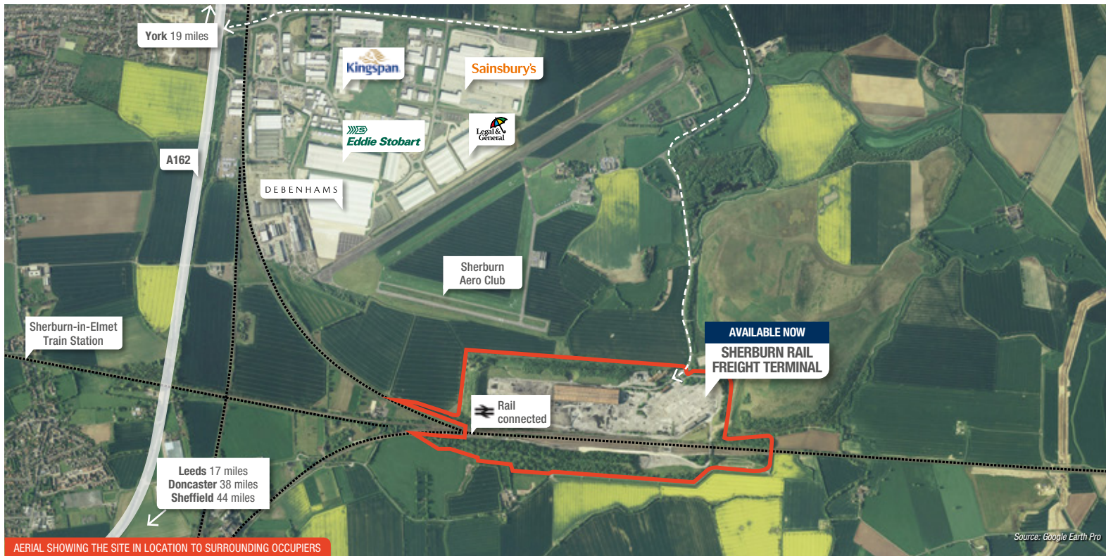
AERIAL SHOWING THE SITE IN LOCATION TO SURROUNDING OCCUPIERS
