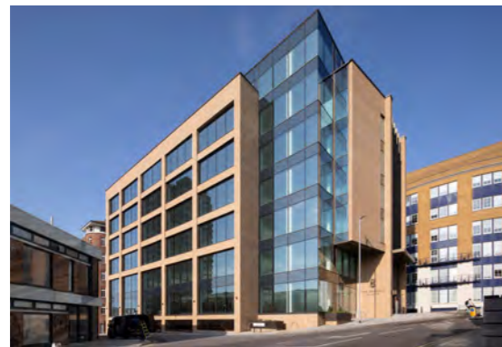
The Brinell Building, Brighton
