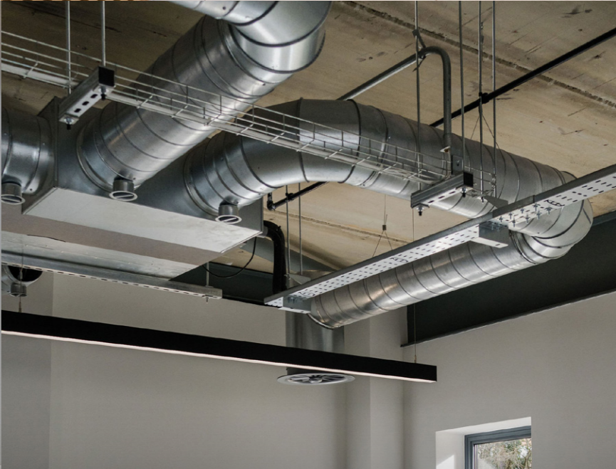
Energy efficient mechanical supply and extract ventilation with heat recovery
