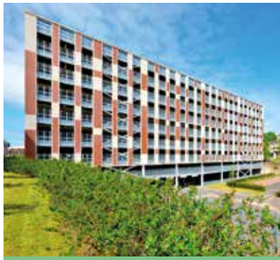
4 Multi-Storey Car Park
