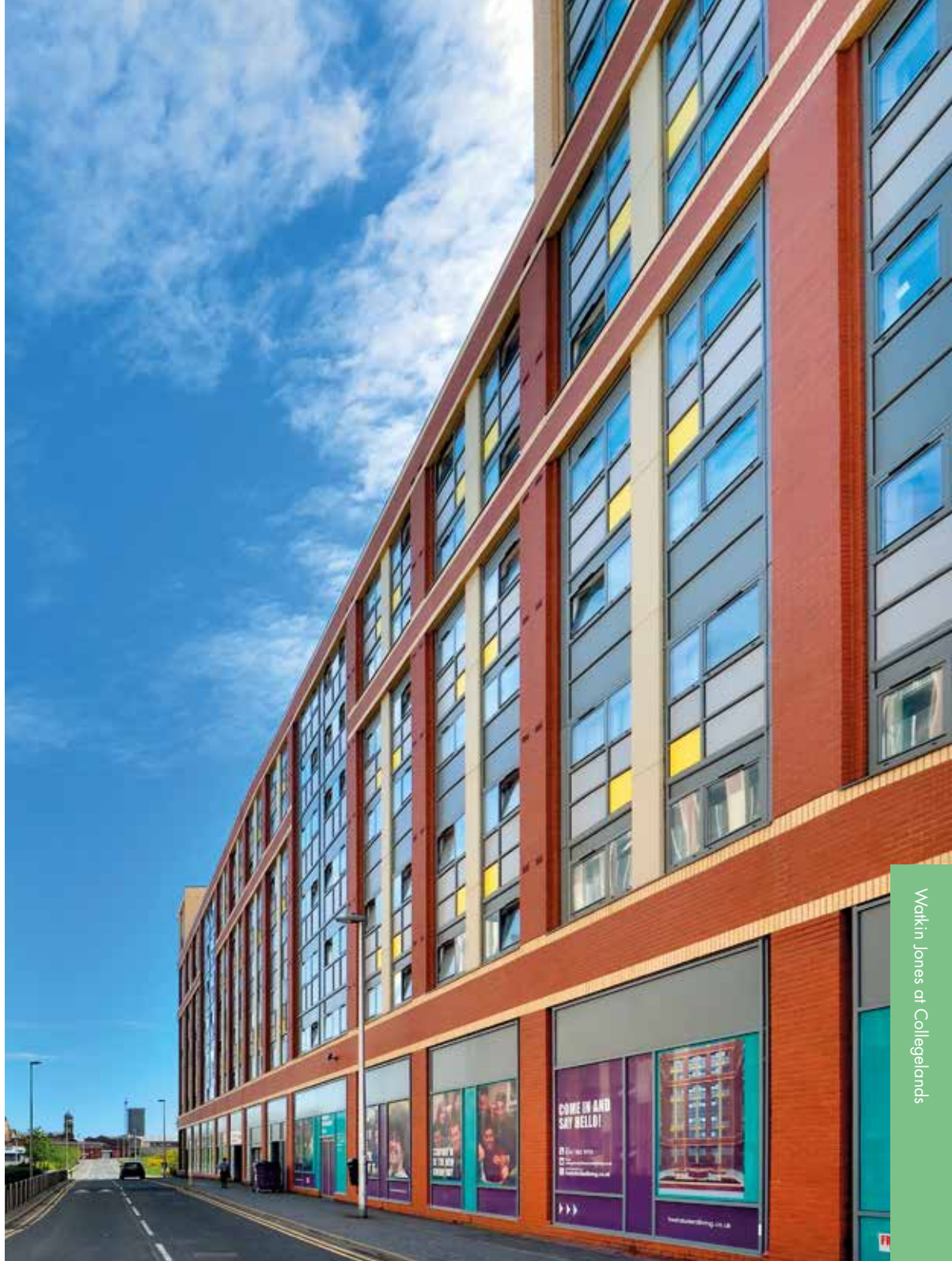
Glasgow City Council new HQ at Collegelands
