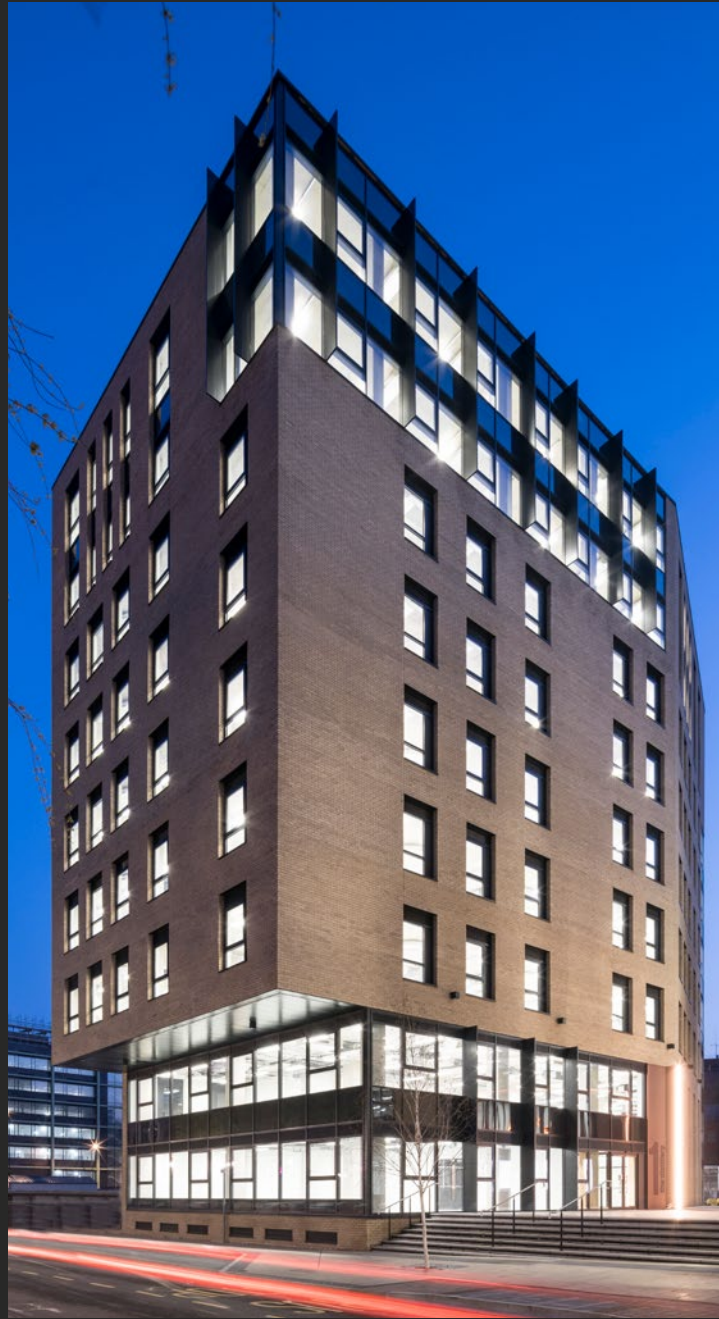
Exterior from Avon Street, entrance and reception
