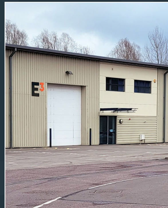
Indicative Image (Unit D Post-Refurbishment)
