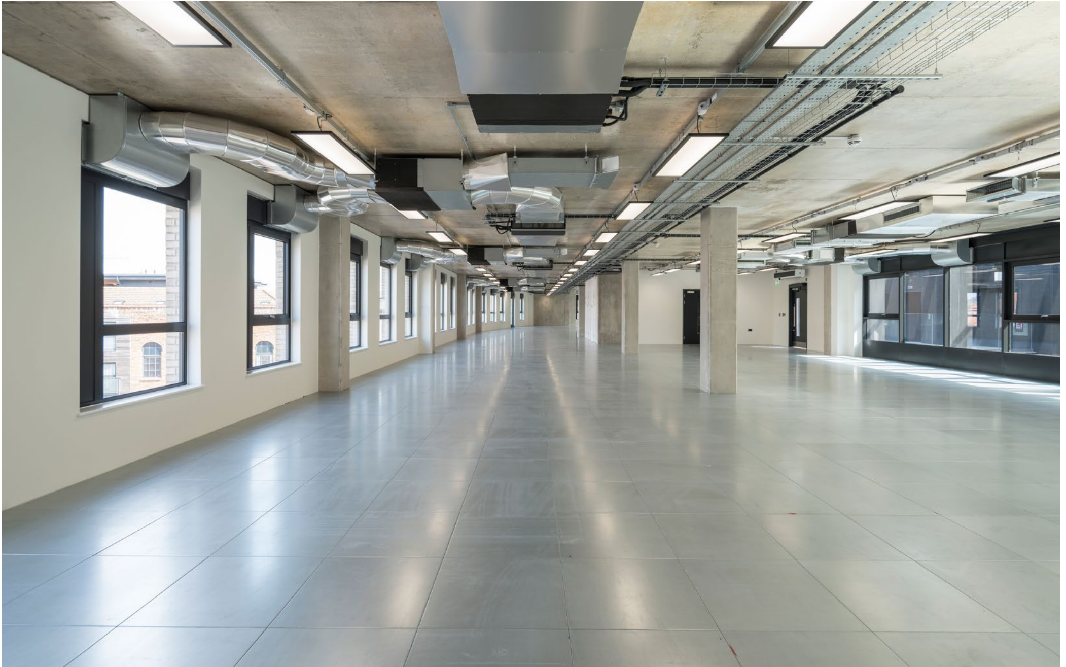
No.2 The Distillery – 3rd floor
