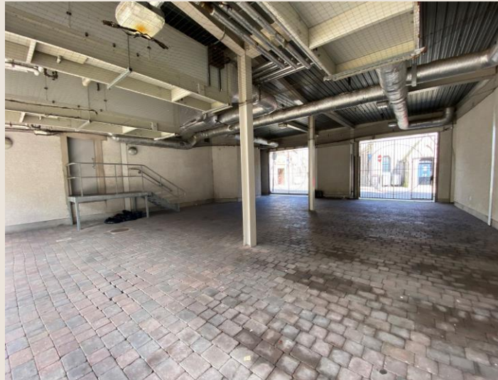
Undercroft car parking accessed from Summer Street
