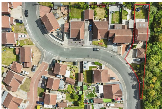
Aerial view of the property
