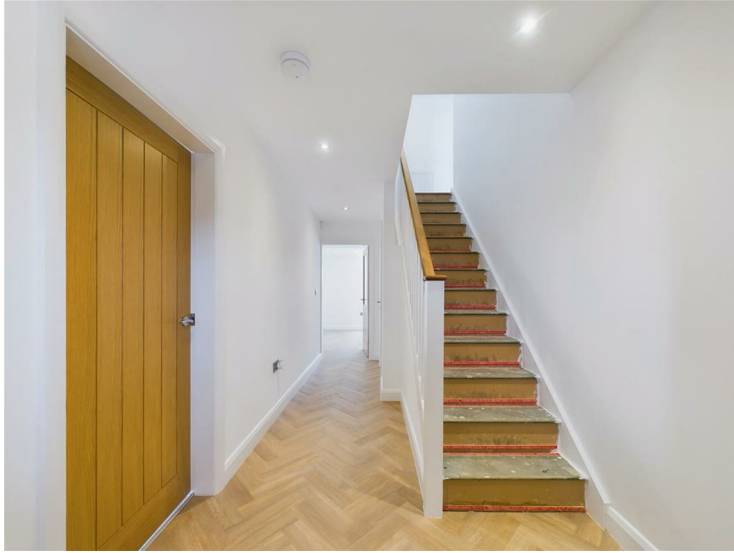
Stairs to first floor landing.
