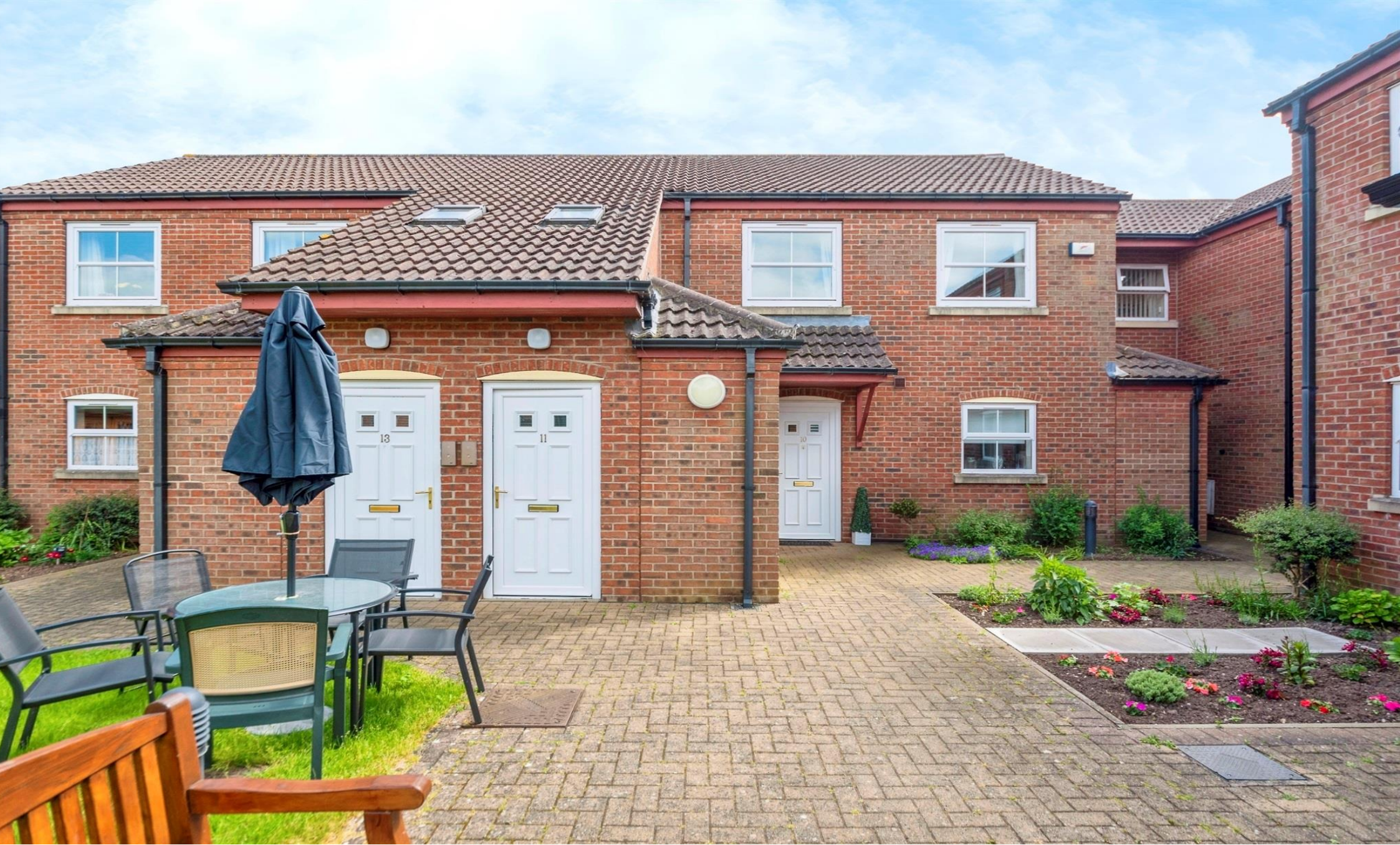
Warwick Court, Balderton, Newark, NG24 3SU
