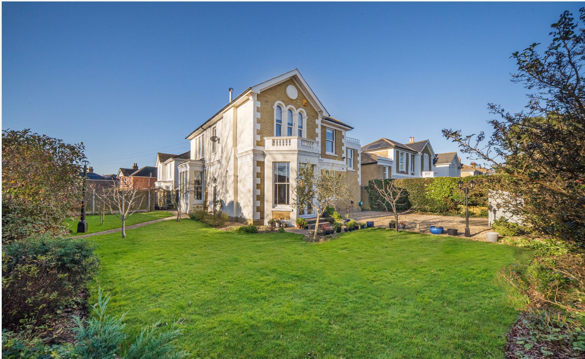
Mannington House 40 High Park Road, Ryde, Isle of Wight, PO33 1BT
