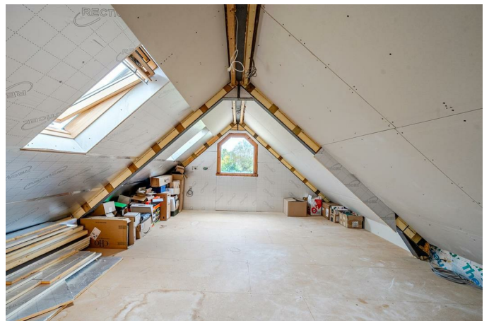
First Floor Bedroom Space
