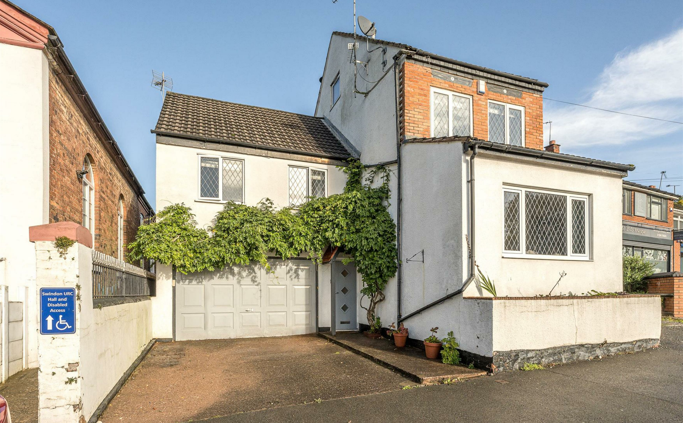
Swindon Cottage, High Street, Swindon, DY3 4NP
