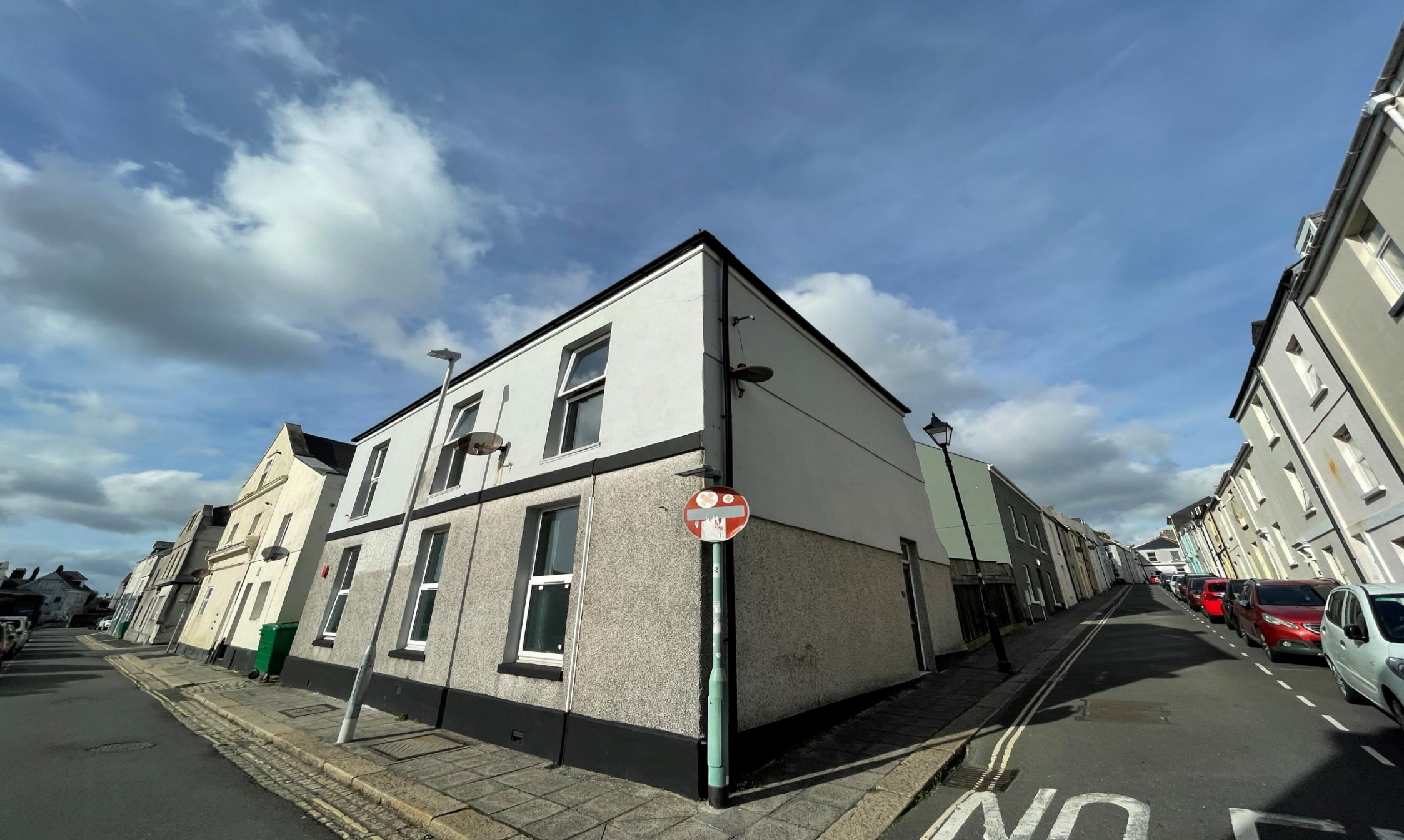
1 Wellington Street & 29 Armada Street Greenbank, Plymouth, PL4 8NB/PL4 8LZ
