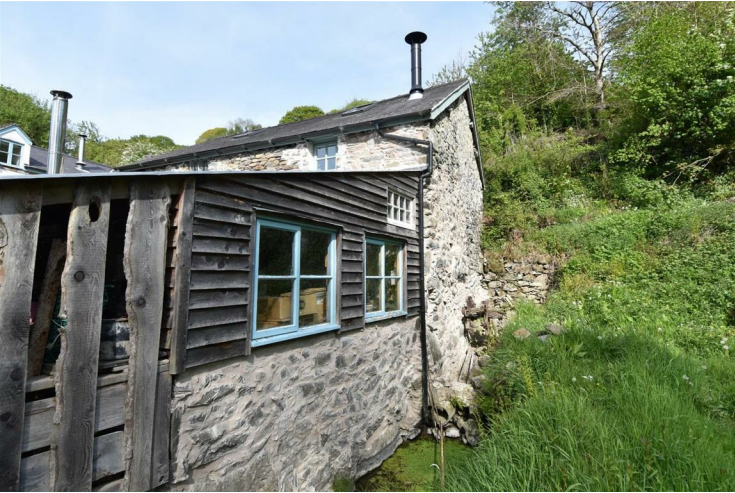
Open fronted log store.
