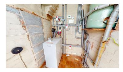
Boiler room housing a Worcester oil fired central heating boiler and electricity meter.
