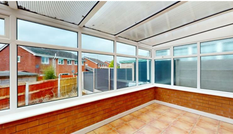
Built on a brick base with UPVC double glazed windows and polycarbonate type roof. Double glazed exterior doors, tiled floor and power points.
