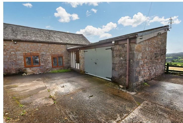
Timber outer doors, useful storage/workshop area, and power and light installed.
