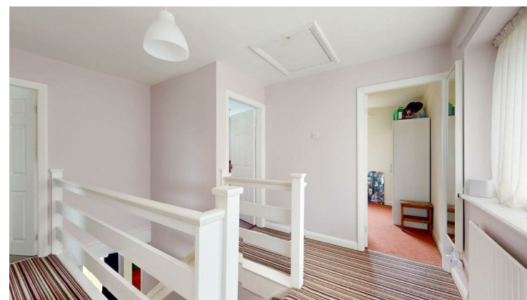
Double glazed window, loft access and radiator. White panelled interior doors lead to all rooms.
