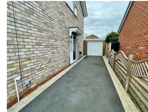
A larger than average garage with an up and over garage door, UPVC double glazed window, UPVC double glazed side personal door, and fluorescent strip light. Integral to the garage there is a wash room and WC.
