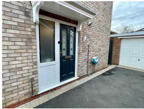
Composite double glazed entrance door with UPVC double glazed side window to the entrance hall.
