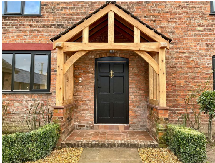
Oak framed entrance porch set on brick piers. Wooden panelled entrance door to the reception hall.
