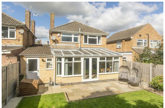
Rear Elevation Picture
