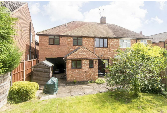
Rear Elevation Picture
